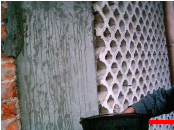
Apply key bonding to concrete surface
